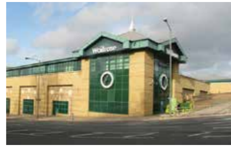
Fig. 1 Photo of the Waitrose store, Bromley South
