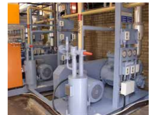
Fig. 2 GEA Grasso 3x310 chiller package in Pick'n'Pay store at Rand Park Ridge
